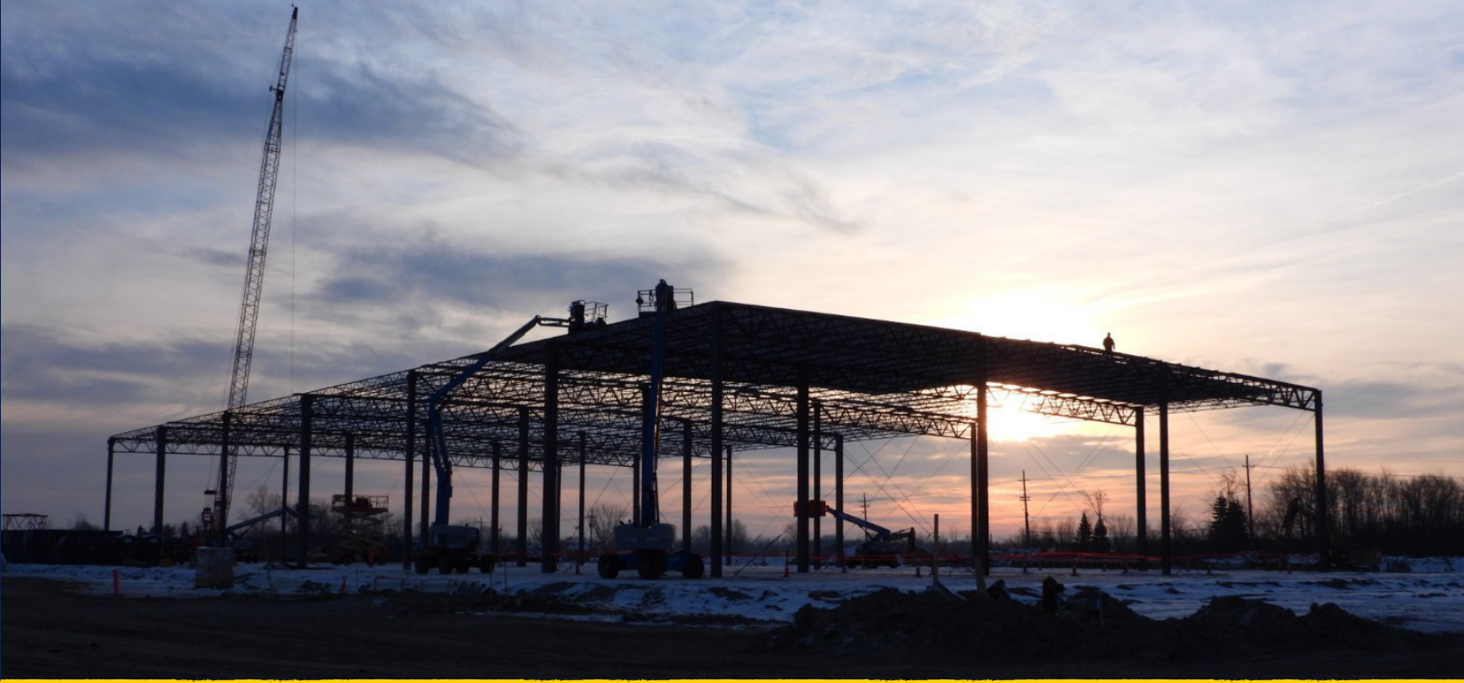
As an AISC Certified Erector, Aristeo ironworkers erected nearly 900 tons of steel for the 265,000 SF Last Mile Delivery Station.
